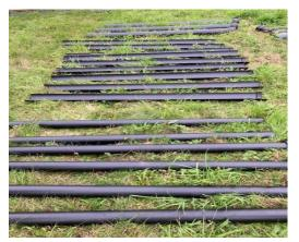
The HCT approved the proposal to fit new cast iron gutters and drain pipes on both walls of the Chapel. The gutters that have now been fitted to new fascia boards along the west elevation are extra deep 6" plain half round gutters with an internal diameter of just under 4". The cast iron hopper draining the roof gully on the north gable has been renovated and fitted to a new oak backboard. The drains have been cleared, and the Chapel is now ready to face the winter.
